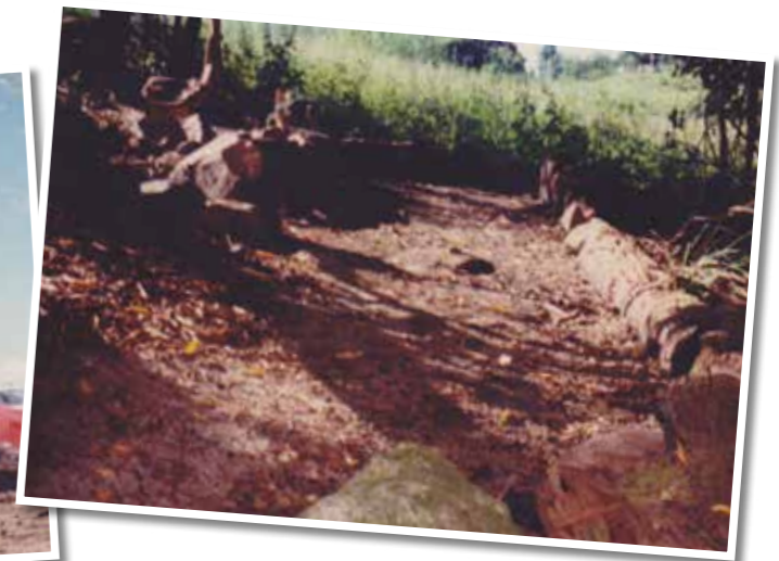
The beginning to the first boardwalk constructed by volunteers down into the wetlands.
