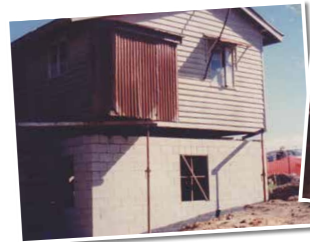
The barracks are taking shape.
